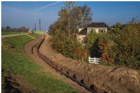
Fig. 3.7 Dyke reinforcement with sheet piles in Wolferen-Sprok [20]
