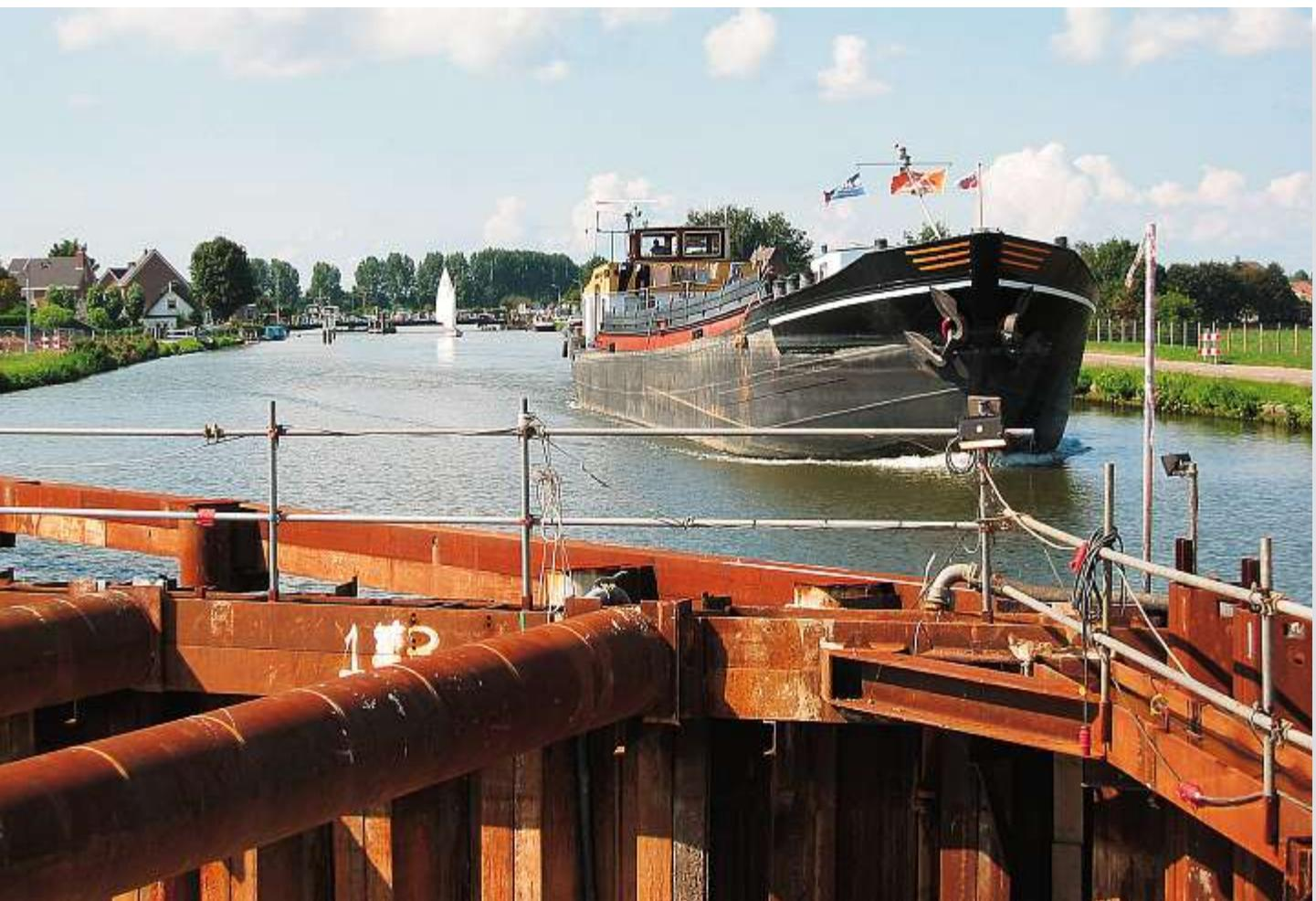
The soil at the site of the Ringvaart aqueduct consists of a Pleistocene sand layer with soft clay and peat layers below, all containing salt water. Water was kept outside the excavation by filling the sheet pile interlocks with the bituminous filler material Beltan that also demonstrated its effectiveness at the Noordrand tunnel site.
