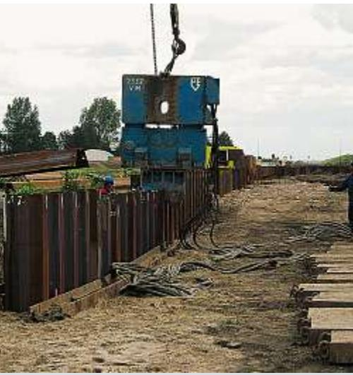
A variable-moment vibrator was used to install and remove the sheet piles. The rig used was capable of driving 15 piles per day and removing 25 per day.
