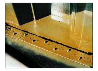
Also a reinforced concrete drag plate is located under the base seal in the base area of the enclosure wall for relocation of the settlements.
