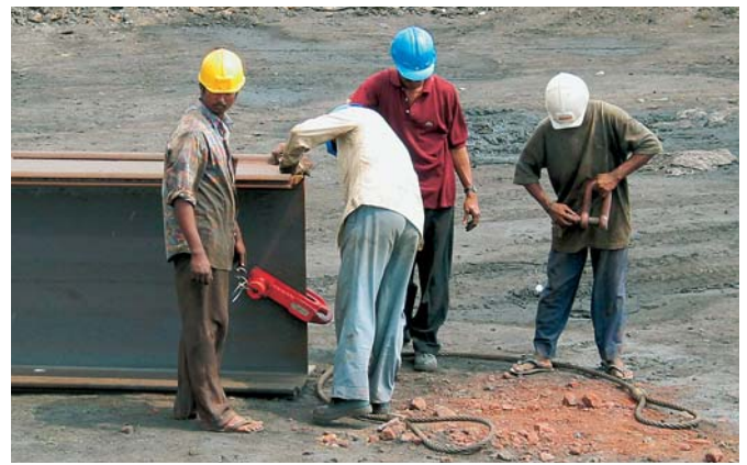
Strong shackles were used to lift the king piles
