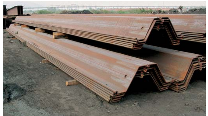
Wooden spacers prevent damage to the stored AZ piles
