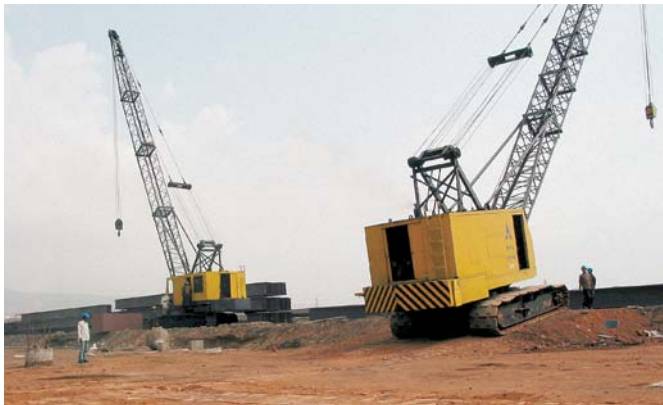
Two crawler cranes lifted hammers and sheet piles into position
