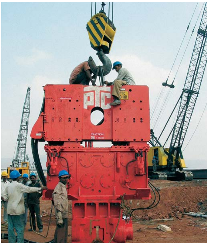
The contractor opted for the PTC 60HD heavy-duty vibratory hammer
