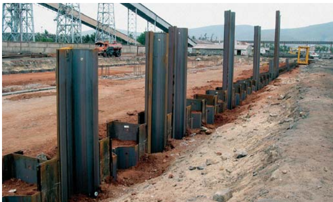
The Indian designer Howe opted for an anchored HZ/AZ combined sheet pile quay wall
