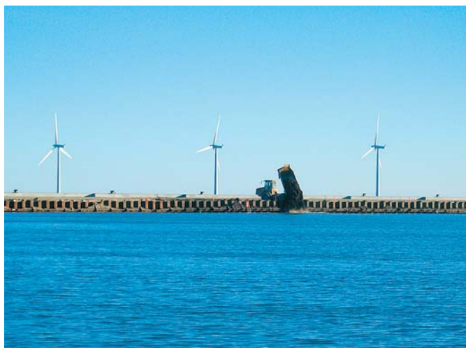
The structure is also an enclosure for dumping soil
