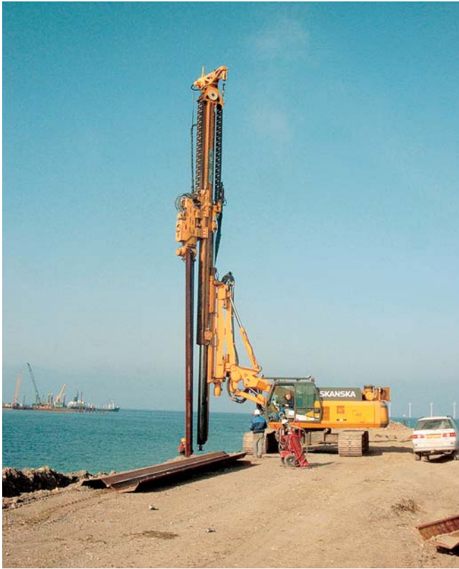
The PU 8 piles were driven into a berm by an excavator-mounted vibratory hammer
