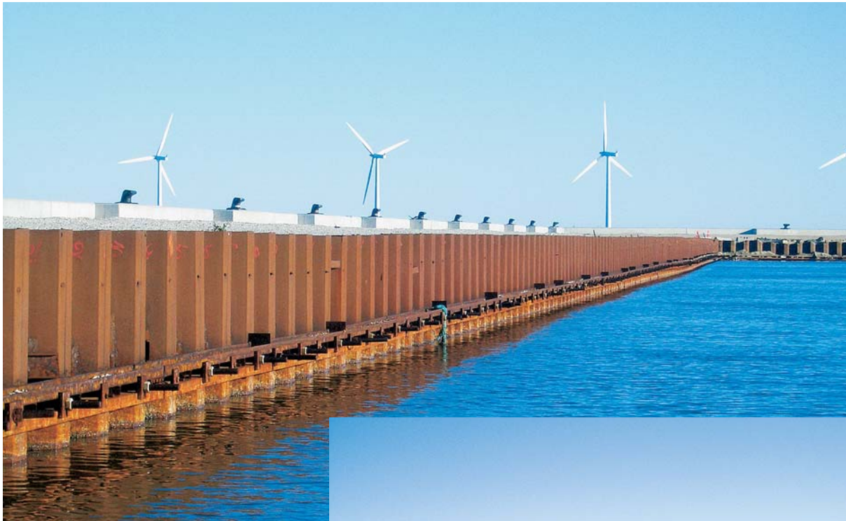
The sheet pile cofferdam forms an impervious barrier for the contaminated soil
