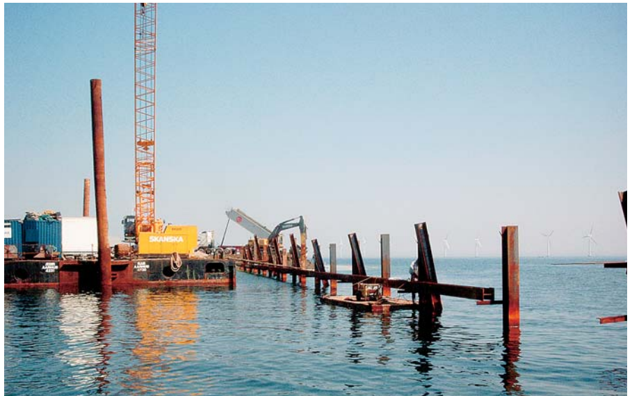
Horizontal beams were used as a driving template
