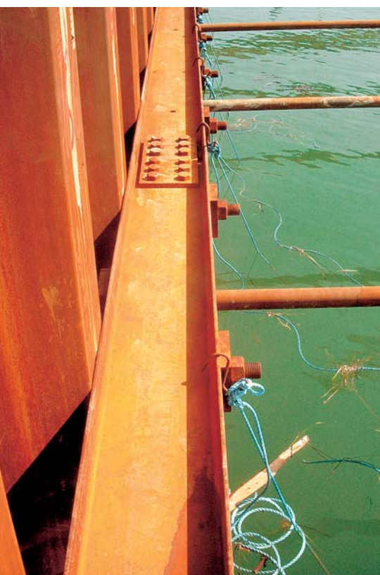
The conventional top tie-rod system includes a waling
