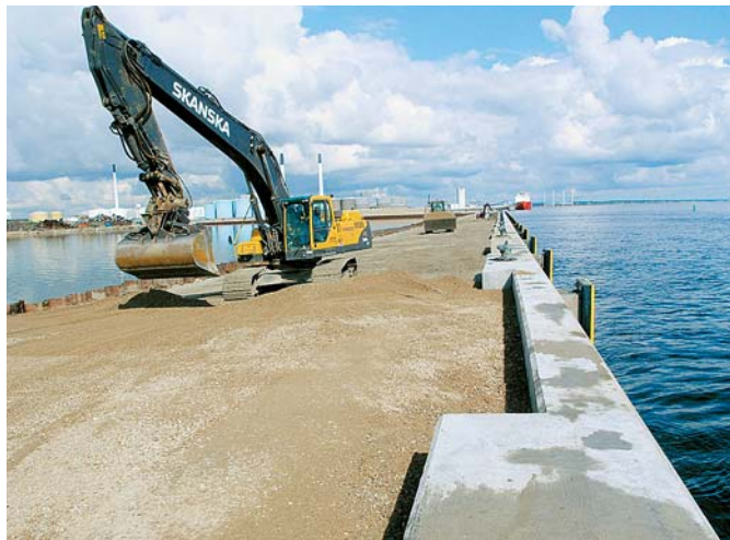
A capping beam fitted with fenders and bollards was placed on top of the sheet piles to finish off the construction
