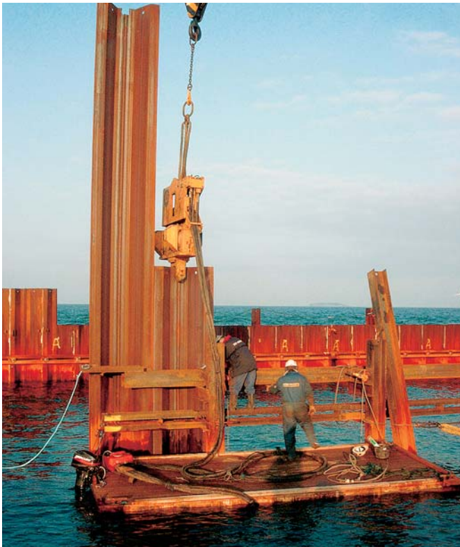
Several barges facilitated the installation of the two cofferdam walls
