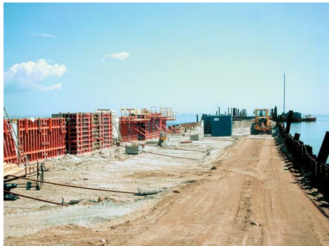
Formwork for the concrete capping beam
