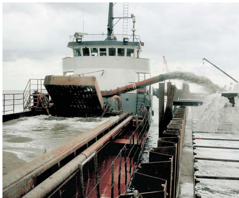
The cofferdam was filled with dredged sand
