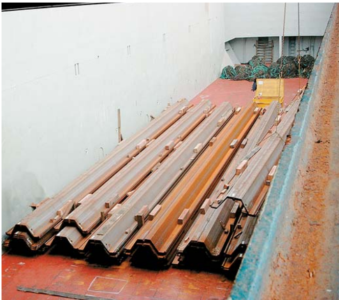
Most of the sheet piles were brought to Prøvestenen by ship
