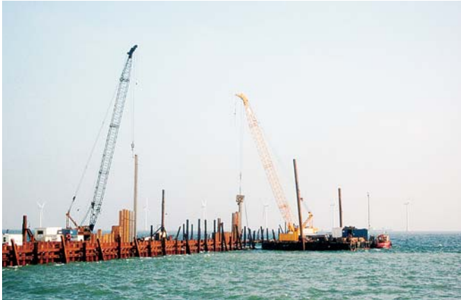
The double-wall cofferdam was installed in open water
