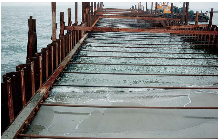
Top steel tie rods of the cofferdam
