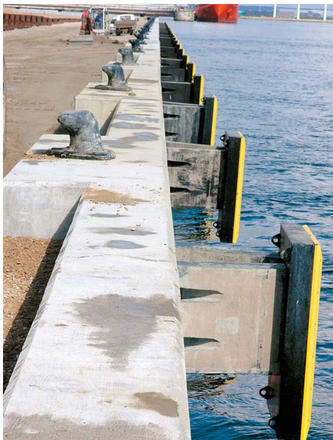
A capping beam fitted with fenders and bollards was placed on top of the sheet piles to finish off the construction
