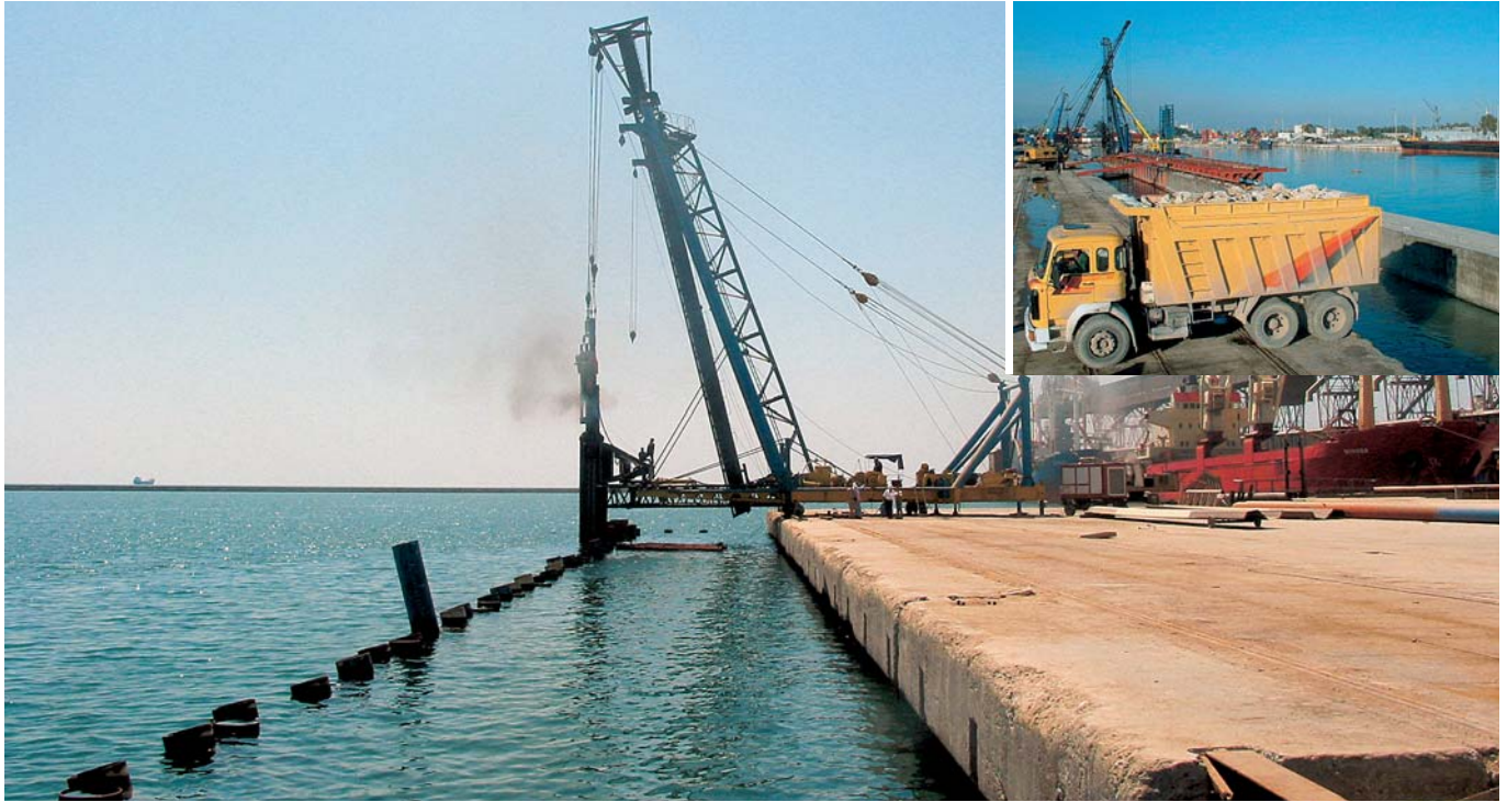
The installation rig used the existing concrete wharf for support
