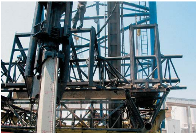
The rubber protectors prevent damage to the coating system during installation
