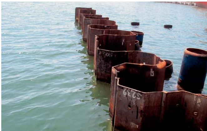
The 624-m sheet pile wall will enlarge the mooring area
