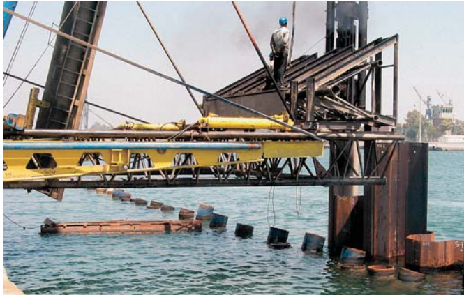
The contractor's template features two steel-tube guiding levels fitted with rubber fenders
