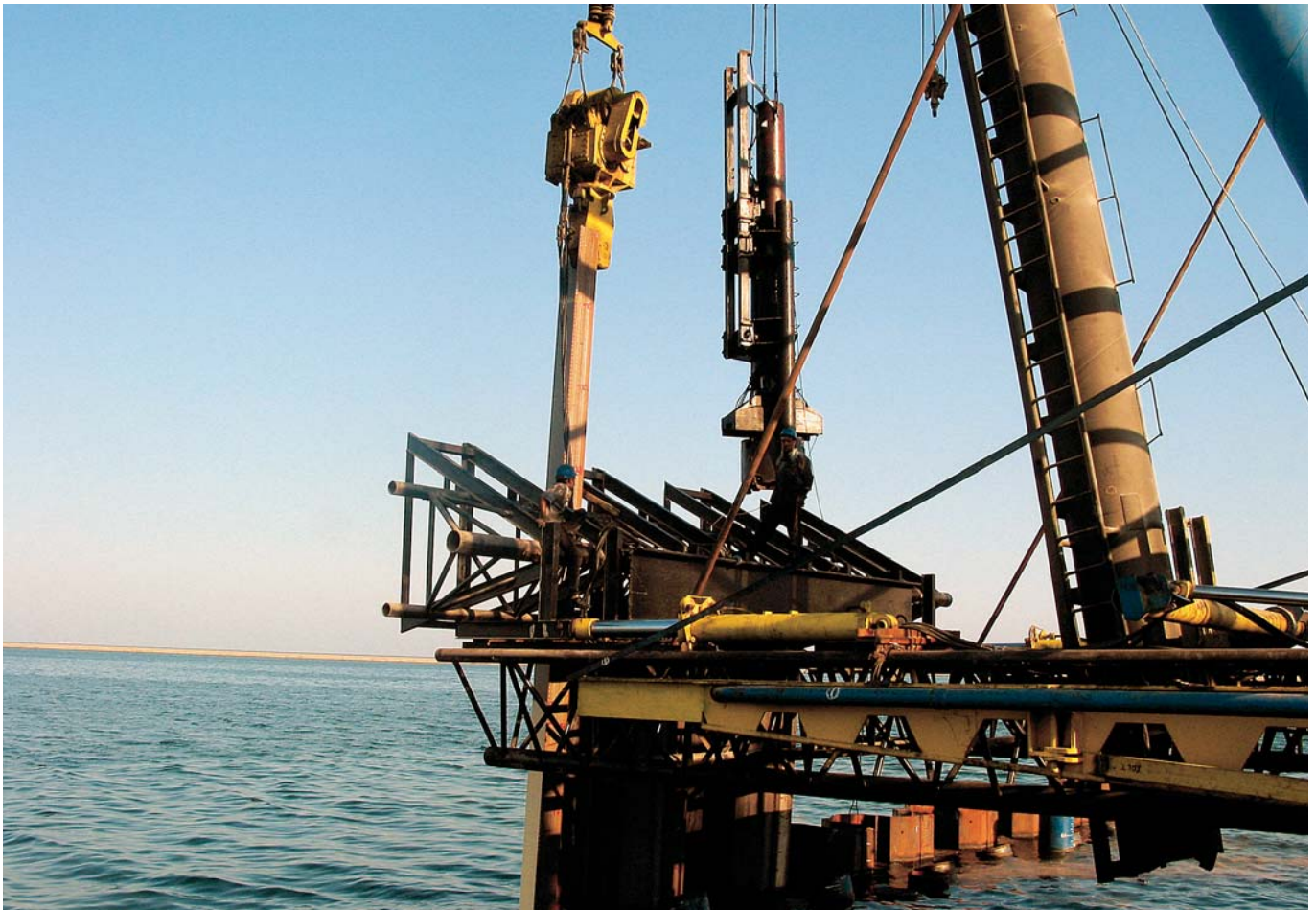
Both the vibratory and the impact hammer were mounted on the specially designed rail-mounted rig
