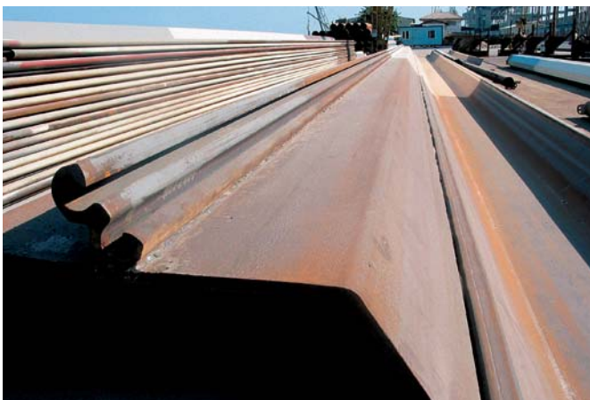
The AU 20 double piles were arranged into a jagged wall using Omega 18 connectors
