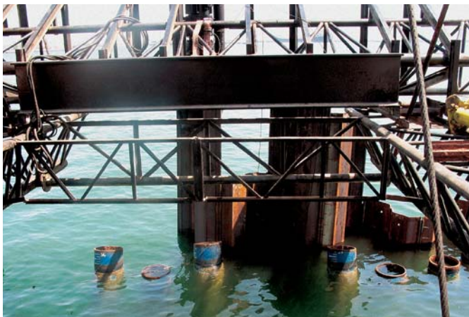
Vertical and inclined batter piles were also installed with the template
