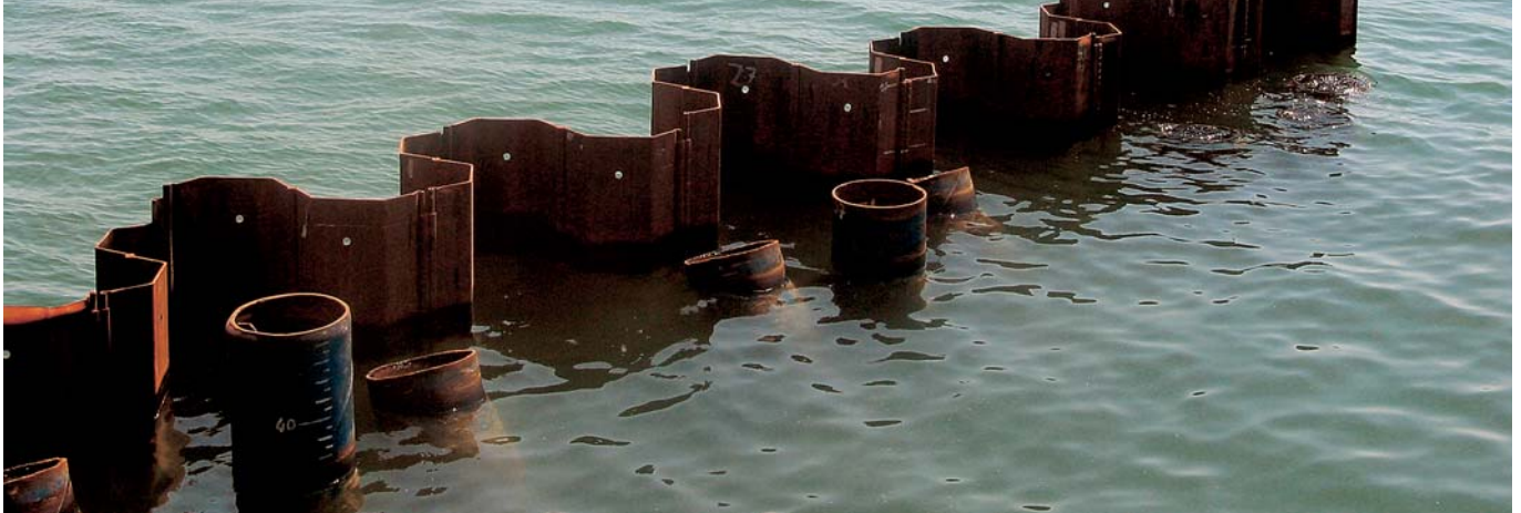
The structural system consisted of a sheet-pile soil-retaining wall, steel crane-foundation piles, and deflection-restricting batter piles
