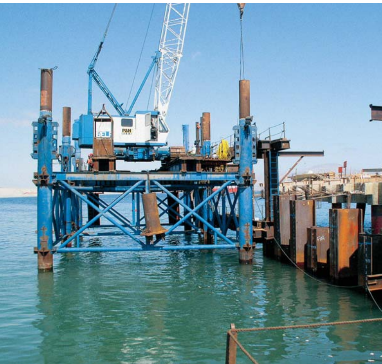
A jack-up barge and a template were used to install the HZ/AZ system
