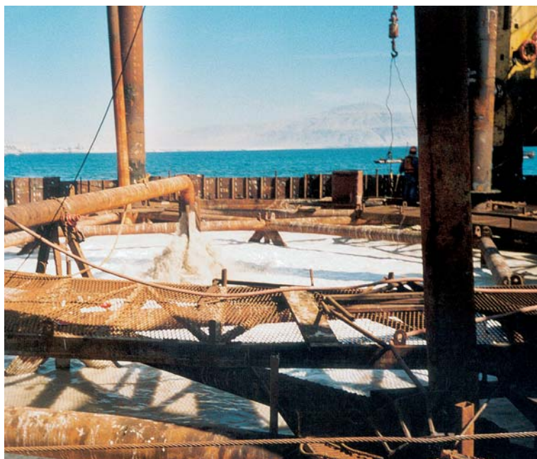
Sheet pile cells are usually filled with locally available sand
