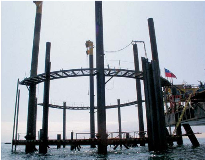
The breakwater is composed of eight cells with a diameter of 24 m
