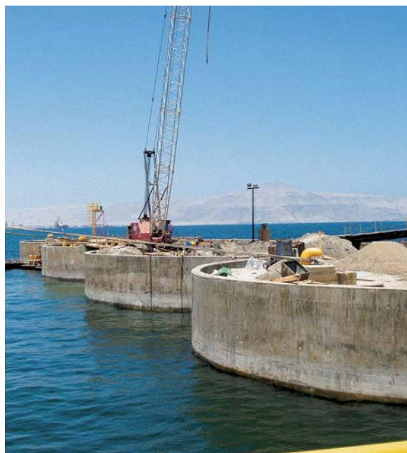
Concrete ring beams protect the cells
