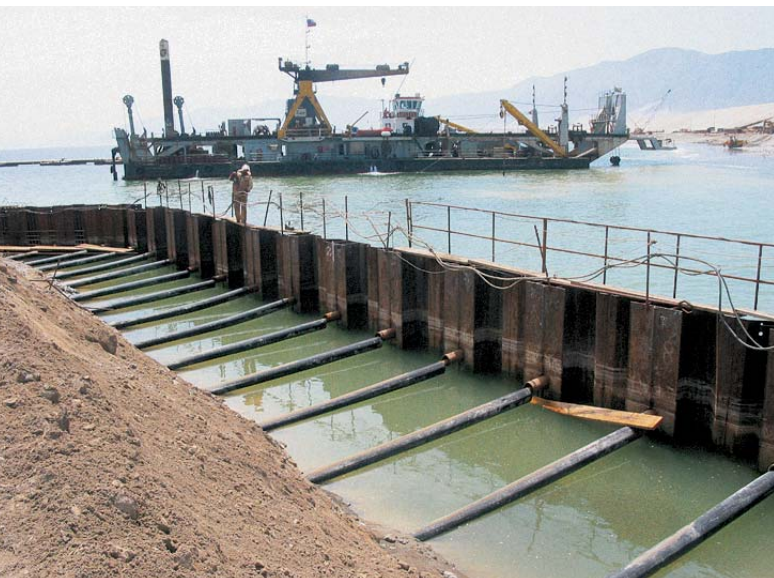
An anchored combined sheet pile wall was chosen as the optimum solution for the quay wall
