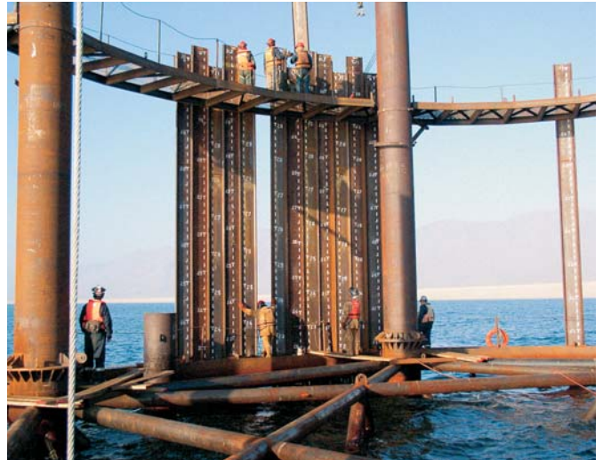
The straight-web sections were installed with the help of a template to form the breakwater cells
