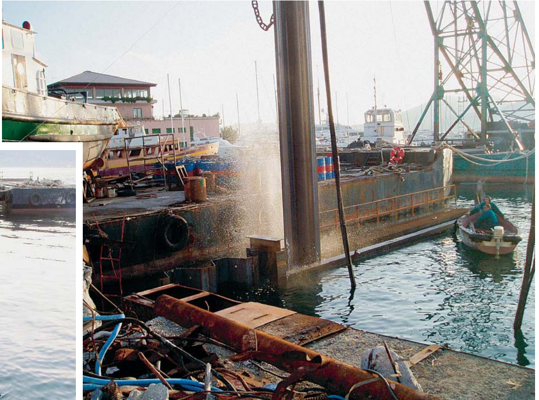
2,600 t of 24-m AZ 36 and 8-m AZ 18 sheet piles were installed
