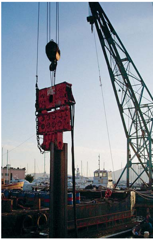
Installation proceeded smoothly with the PTC vibratory hammer and the driving template
