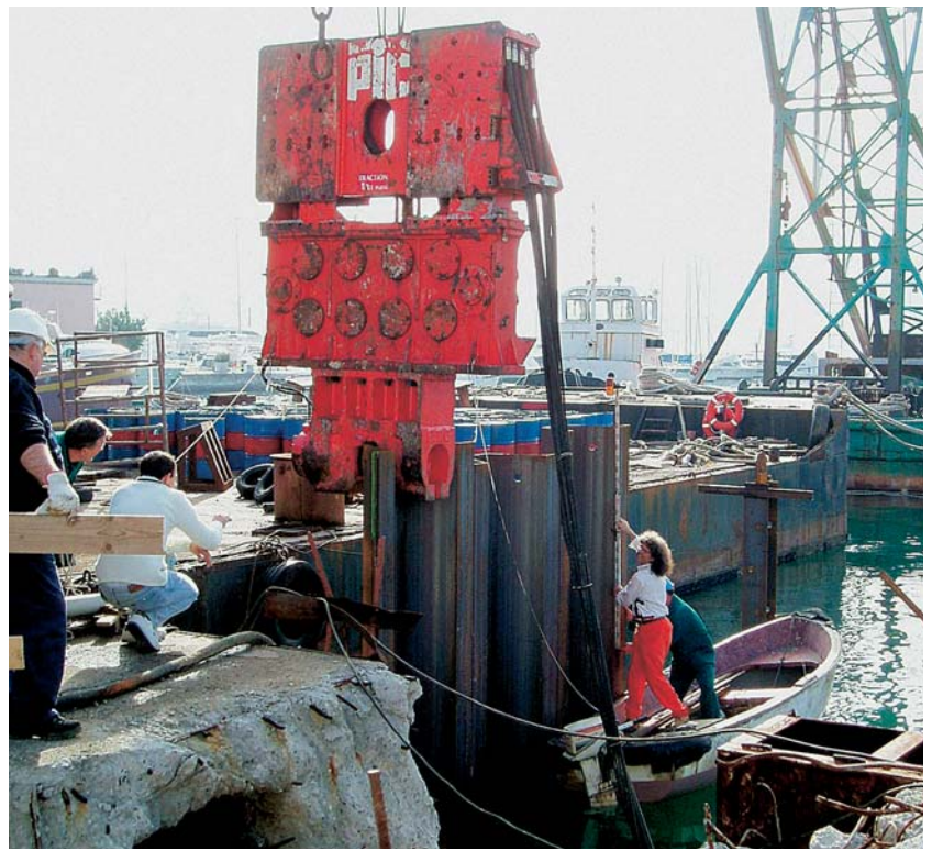
Installation proceeded smoothly with the PTC vibratory hammer and the driving template
