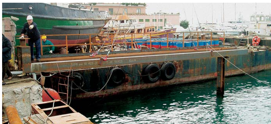
The new 400-m pier will be completed by 2006 using AZ 36 and AZ 18 sheet piles
