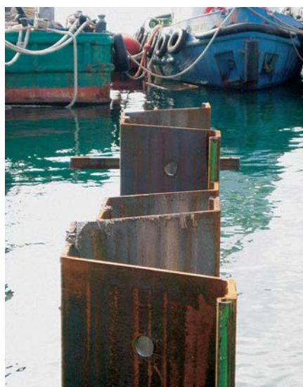
A template was used for the installation of the AZ piles
