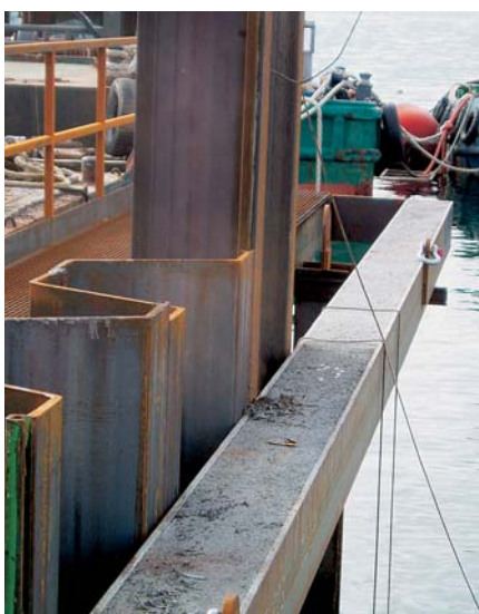
A template was used for the installation of the AZ piles
