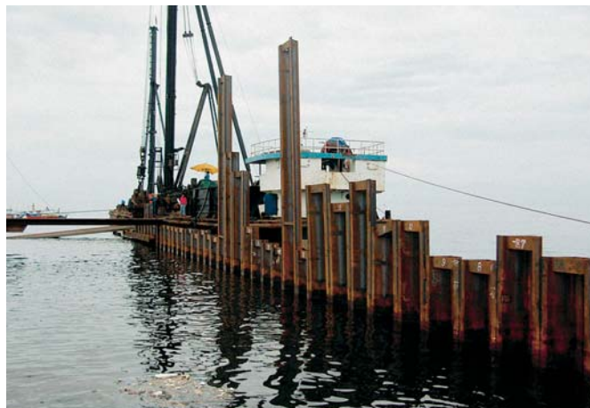
AZ double piles up to 21.5 m long were installed with barge-based driving equipment
