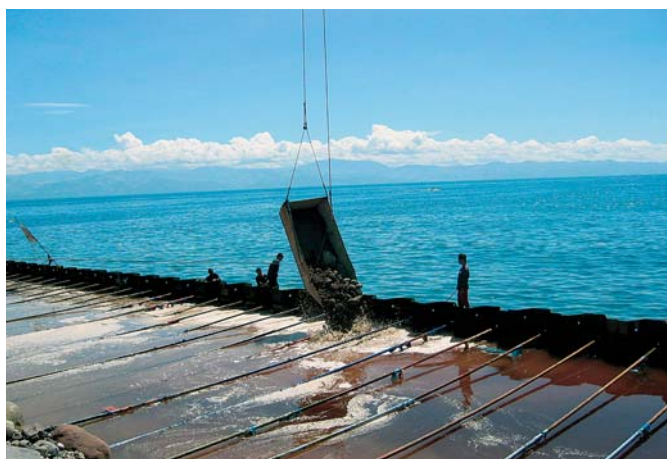
The area behind the AZ wall was backfilled carefully so as not to damage the tie rods
