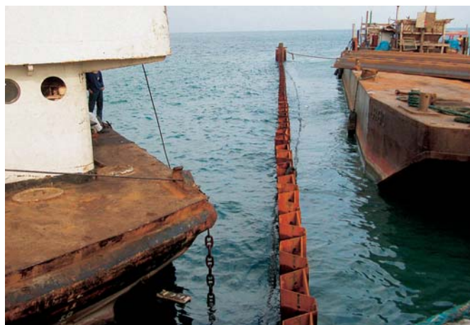
The two wharves were built using 380 AZ 34 double sheet piles as well as 80 AZ 26 double sheet piles
