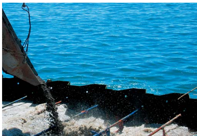
The area behind the AZ wall was backfilled carefully so as not to damage the tie rods
