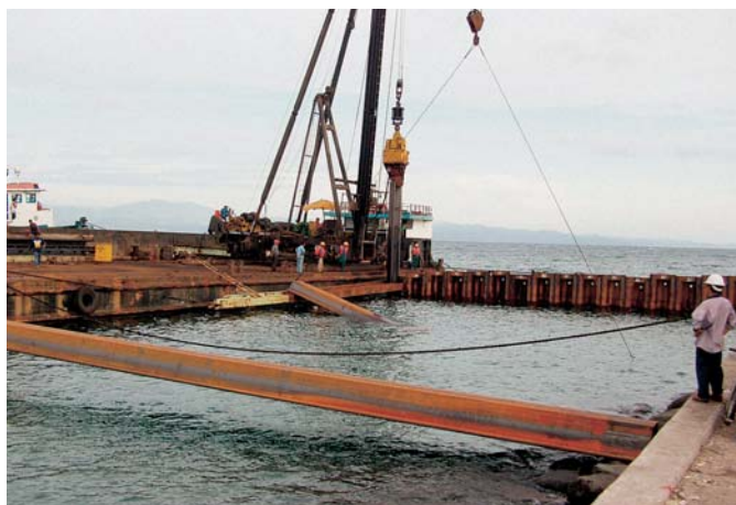
The two wharves were built using 380 AZ 34 double sheet piles as well as 80 AZ 26 double sheet piles
