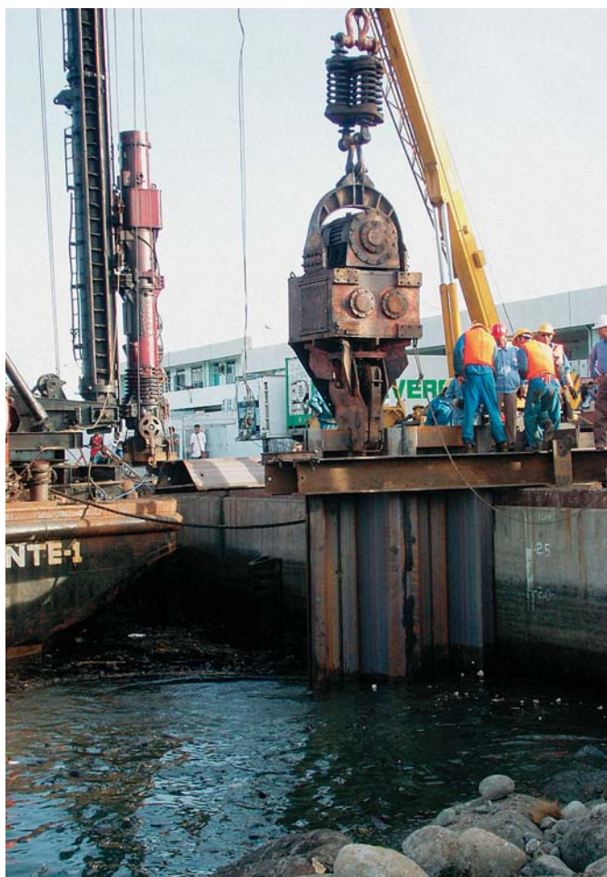
A vibratory hammer was used first; a diesel hammer then completed the installation process
