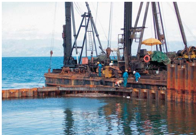
AZ double piles up to 21.5 m long were installed with barge-based driving equipment
