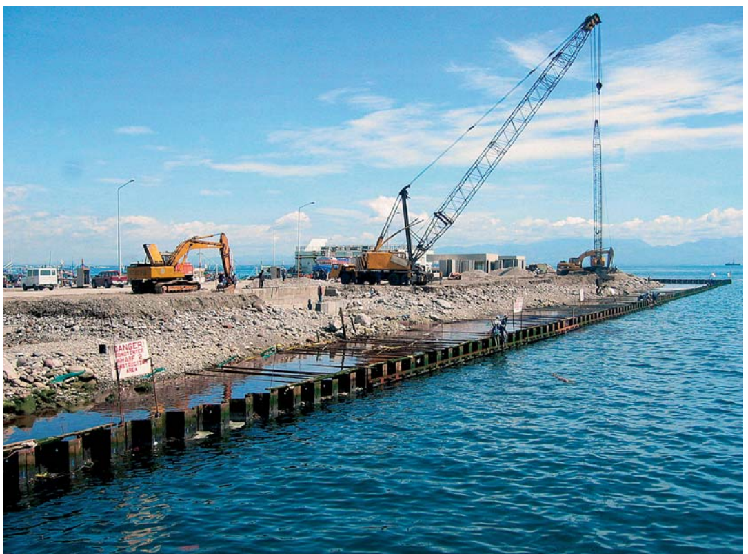
Two AZ sheet pile quay walls were required by the growing tuna fishing industry
