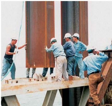
A two-level rigid template ensured the verticality of the king piles
