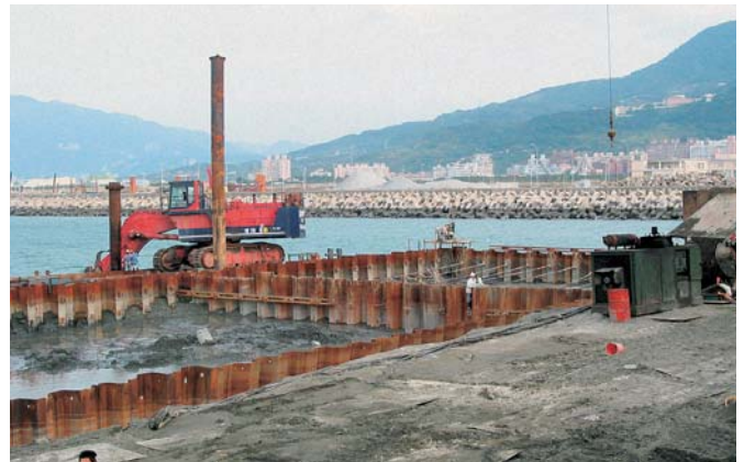
A large excavator was used to backfill the area between the main and anchor walls
