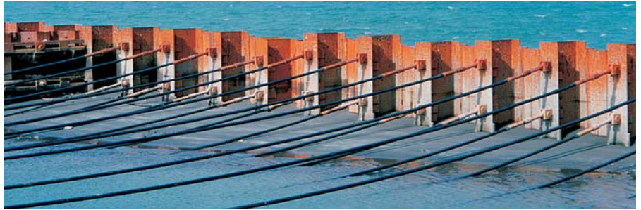
Two layers of tie rods connected main and anchor walls
