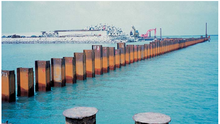
The wall lengths of Quays 13, 14 & 15 are 150 m, 300 m & 250 m
