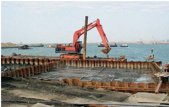
A large excavator was used to backfill the area between the main and anchor walls
