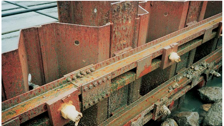
Two levels of load-distributing walings were installed
