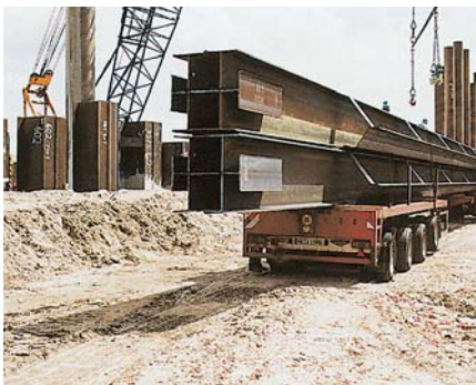
The joined sheet pile elements were delivered just in time
