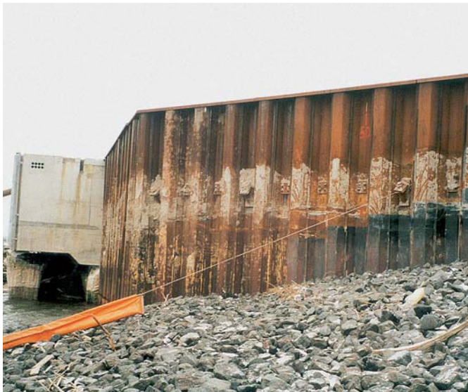
A sheet pile wall finishes off the terminal at both ends
