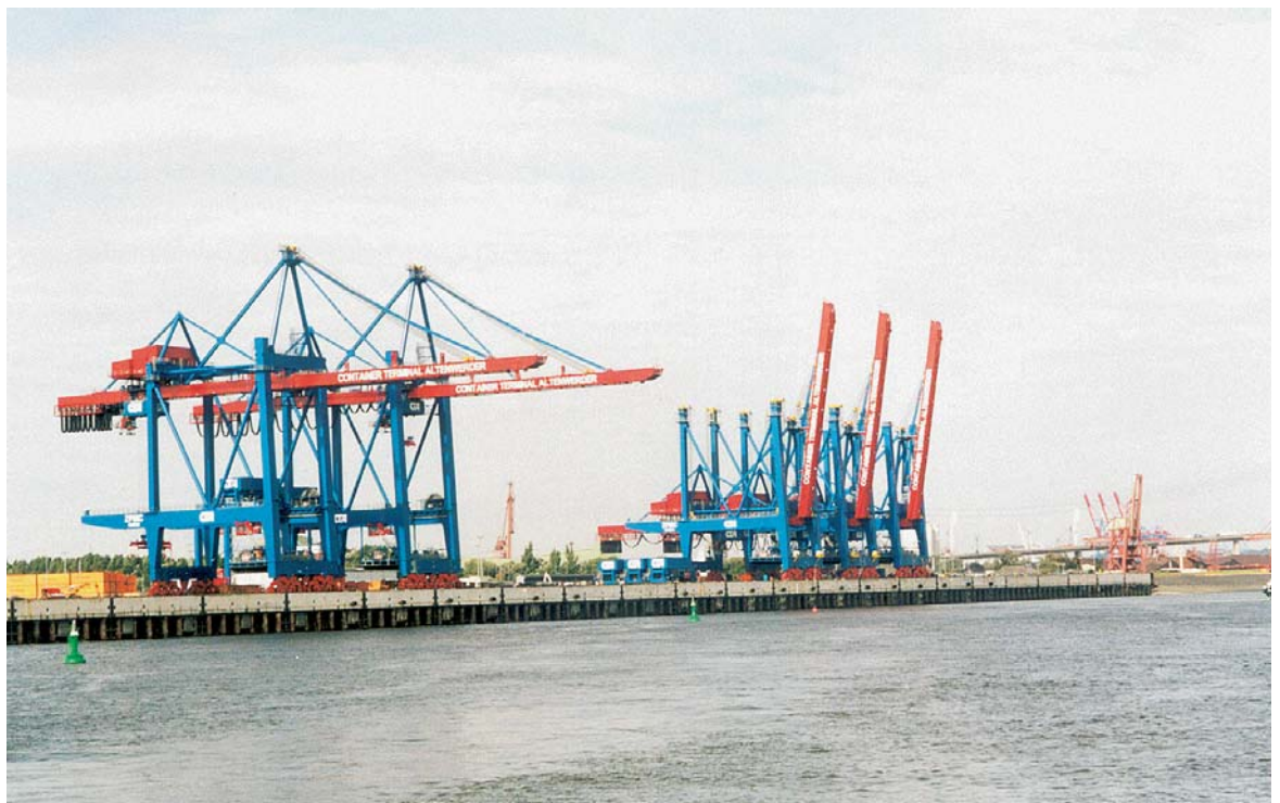
The new Altenwerder CT will handle 1.9 million TEU per year
